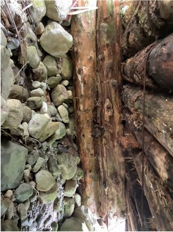
Right Bank Abutment when facing downstream
