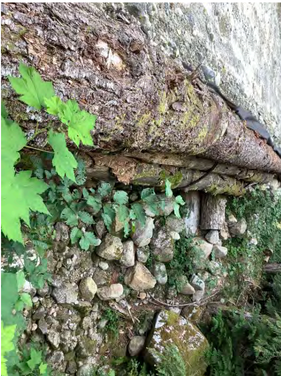
Downstream Profile - note conk in outside stringer
