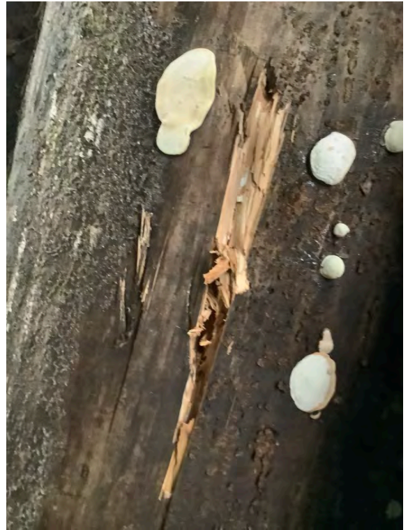
Typical stringer condition
