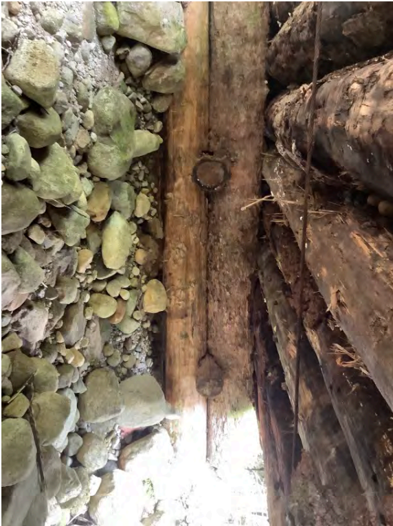
Right Bank Abutment when facing downstream
